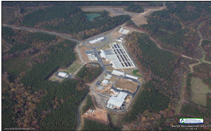
Figure 1- Western Wake Regional Water Reclamation Facility
